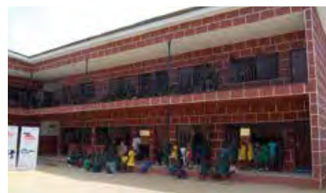
Renovation of Bonny Camp School by the Personal Banking Division.
